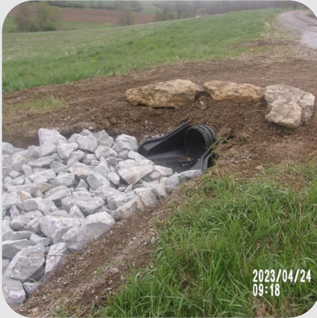
Short Cut Road Drainage project, April 2023. Poor road drainage along the roadway caused yearly maintenance required to keep the road open during the wet season. Pictured is the outlet of one of the 9 new cross pipes being installed along with 10 ditch outlets to manage stormwater more efficiently.
