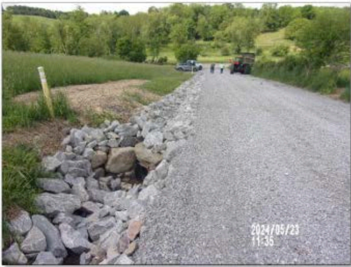
Brady Road Drainage Project: The Brady Road Dirt and Gravel Project raised a portion of the entrenched roadway, replaced 3 cross pipes and added 2 new pipes and installed new inlets and outlets. 770 Feet of Riprap lined ditches were added. 360 Feet of 18” HDPE Storm Pipe was used for the project.
