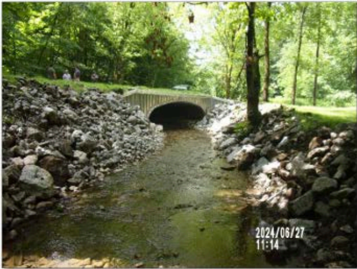
McCready Road Culvert #1: The McCready Road Dirt and Gravel Project replaced a failing multi-pipe culvert with an open bottom arch culvert/bridge. This was the 3rd culvert replacement on McCready Road. Bank stabilization was also completed as part of the project and the roadway was also raised to meet the bridge height.
