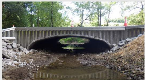
Looking downstream, new structure with low flow channel and proper alignment
