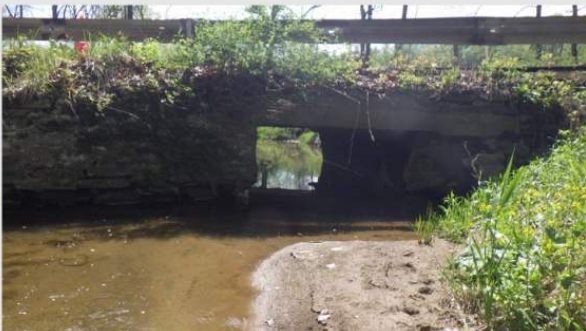
Looking downstream, old bridge with eroding banks due to improper bridge size and alignment.
