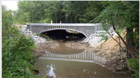
Looking upstream - new structure with grade control structure at the bottom of the photo
