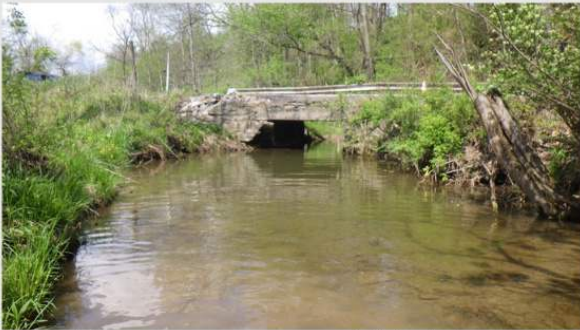
Looking upstream, old bridge with large scour pool
