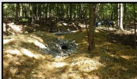
Beech Knob Road: This Dirt and Gravel Project added 8 new cross drains with headwalls and R6 riprap energy dissipators at the outlet. 400' of riprap-lined ditches were added, along with re-establishing 1,481' of roadside ditch. 4 new turnouts were also installed. 240' of 15" HDPE storm pipe was used for this project.
